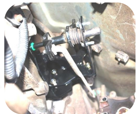
Figure 9 Transfer Case Linkage Installed
